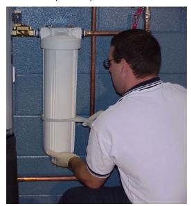
Photo 6. Disassembling the External Prefilter Housing
